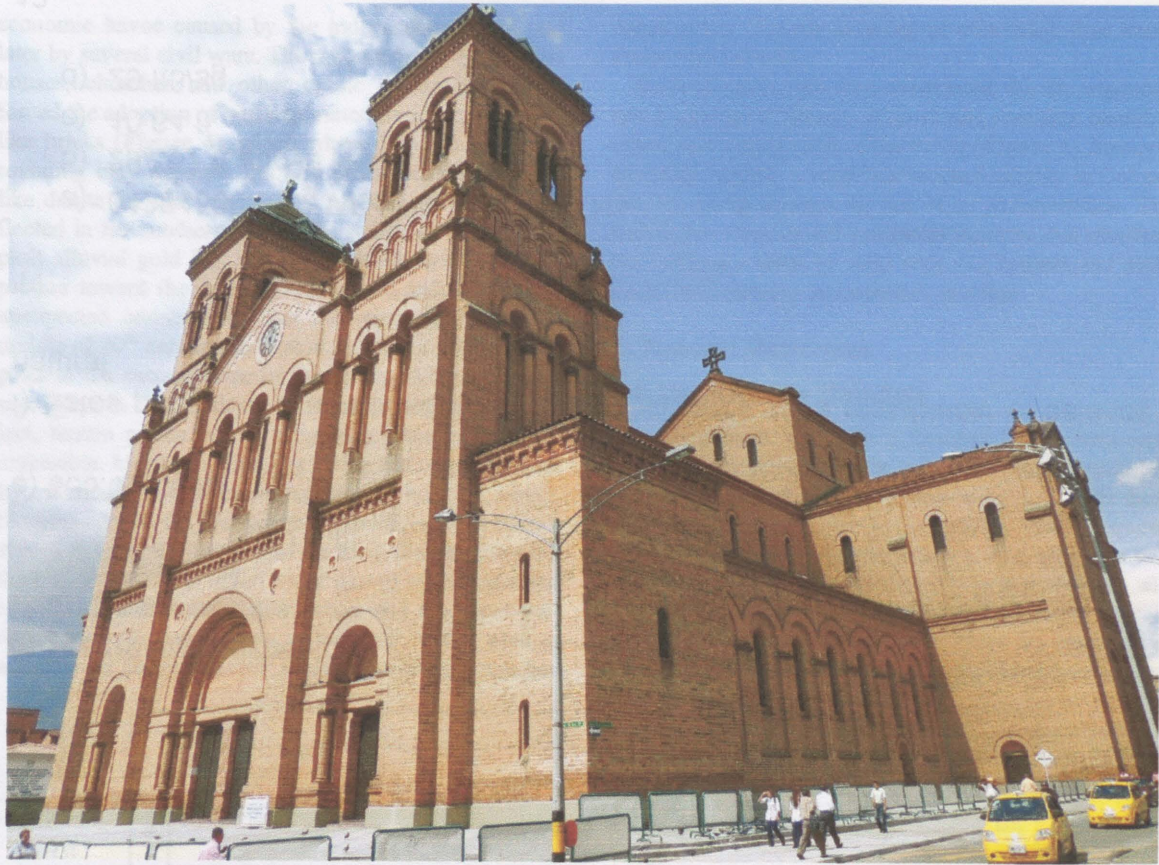
Figure 4. Medellin cathedral, one of the largest brick buildings in the world.
